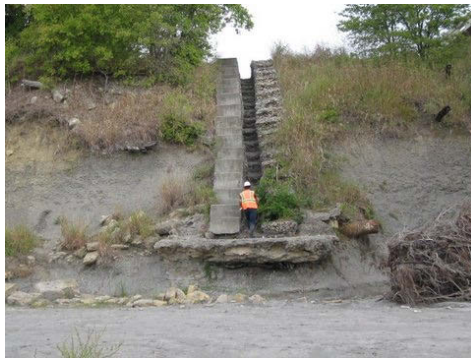
These stairs were made for giants!
